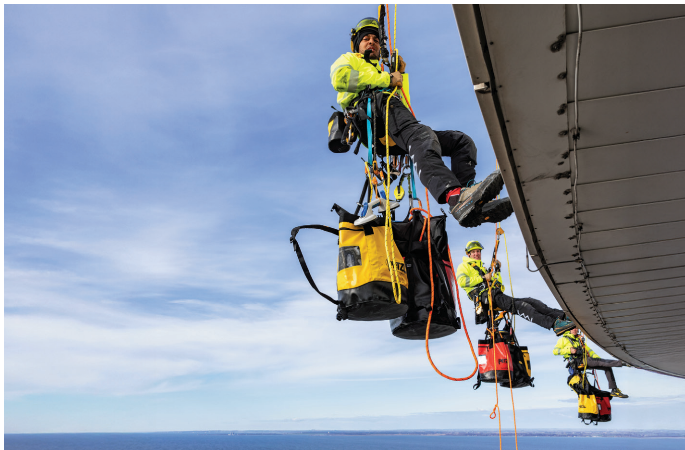
Window cleaning Rope access Sweden © 2023 Petzl Distribution - Lafouche - VYN AB - Turning Torso
