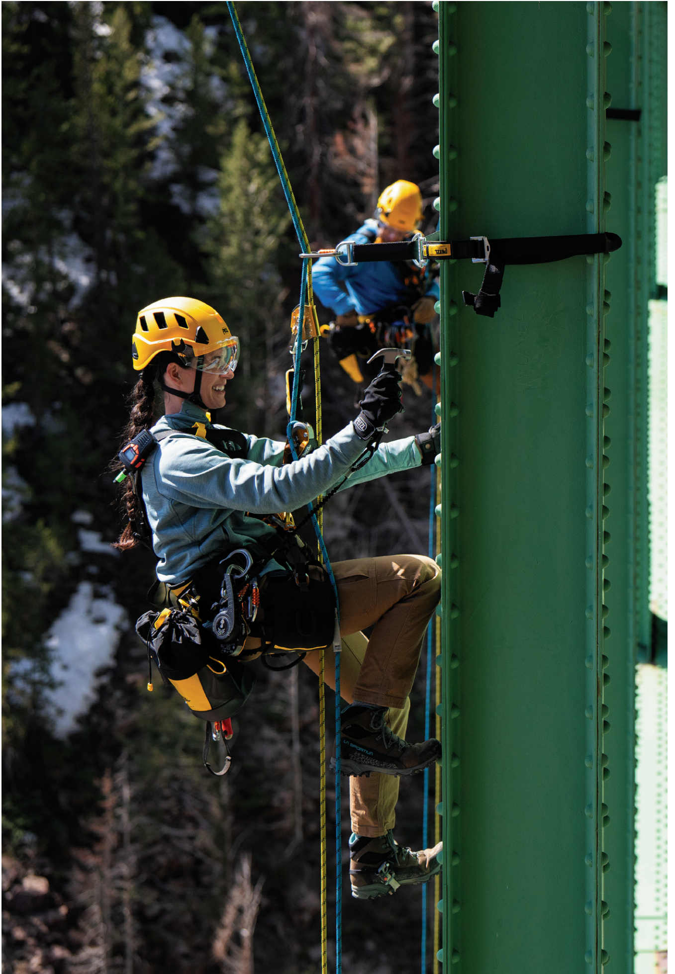
Bridge Inspection Red Cliff Bridge Colorado USA © 2024 - PETZL DISTRIBUTION - Latouche
