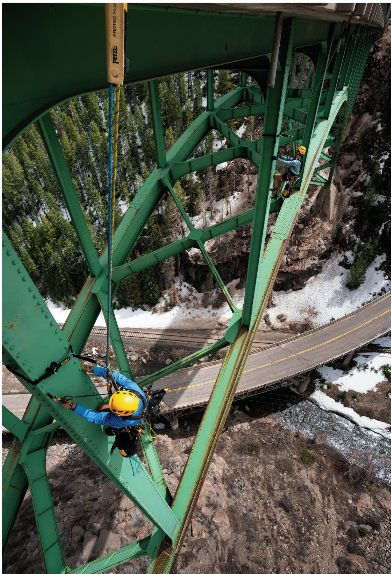
Bridge inspection Red Cliff Bridge Colorado USA © 2024 - PETZL DISTRIBUTION - Lafouche
